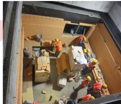
Image 3: Brick Lining of the Side Walls of the POT
