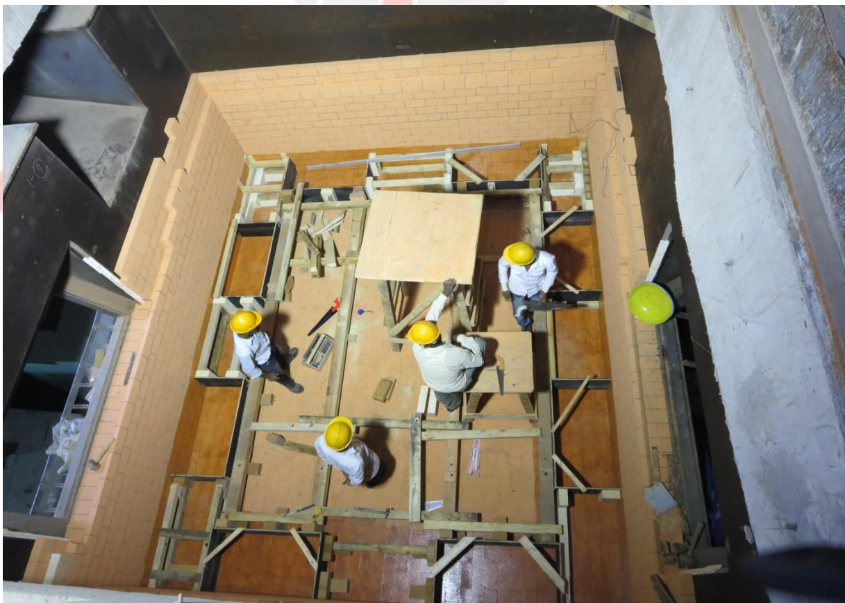
Image 4: Shuttering for the Outer Layer
