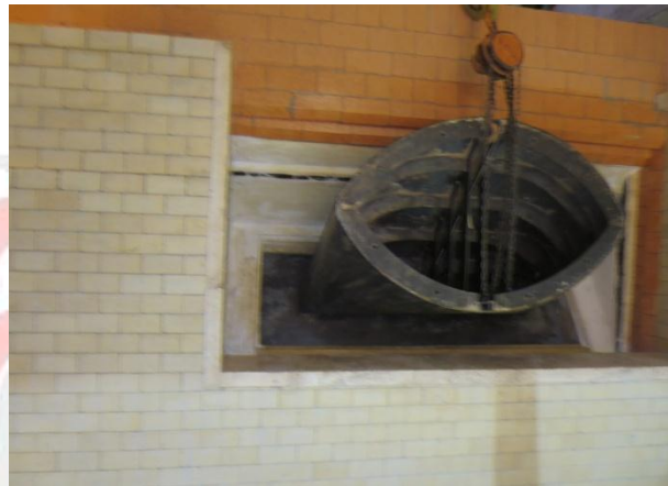
Image 9: Farma Fixing for the Throat Casting
