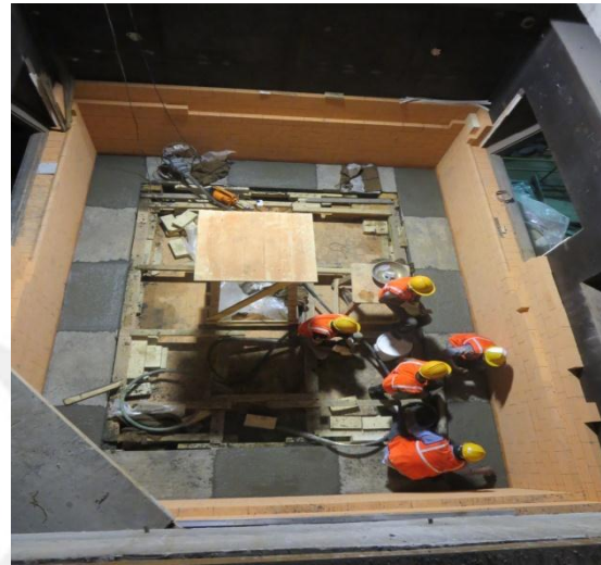
Image 6: Casting of the remaining 8 parts
