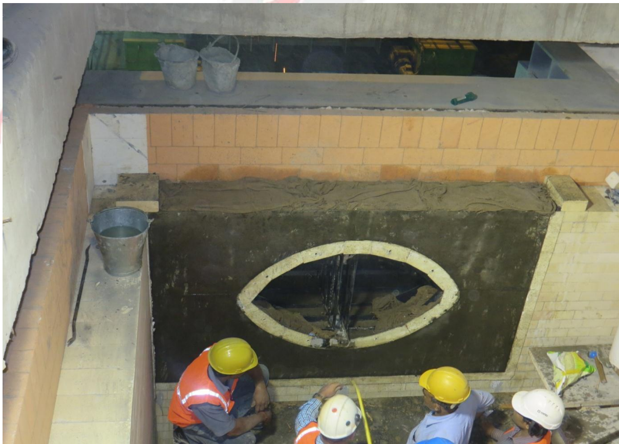
Image 10: Completed Casting of the 2 nd Throat
